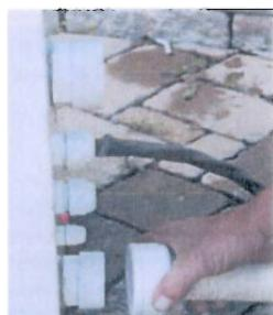
2. Plug the bottom hole with a plug and then, rinse the inside of the exchanger by inserting a garden hose in the top orifice. Leave The water drains for 30 to 45 seconds.
