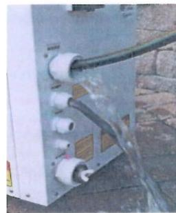
3. Remove the bottom cap and suck up the remaining water in the exchanger using a vacuum cleaner (Shop Vac) by inserting the hose into the bottom port while partially blocking the top orifice with your hand
